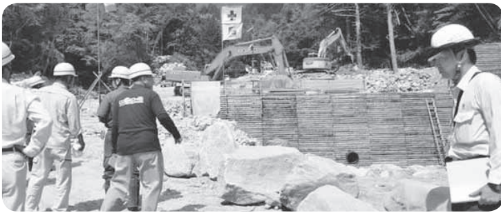
▶芦間川災害復旧工事現地視察
